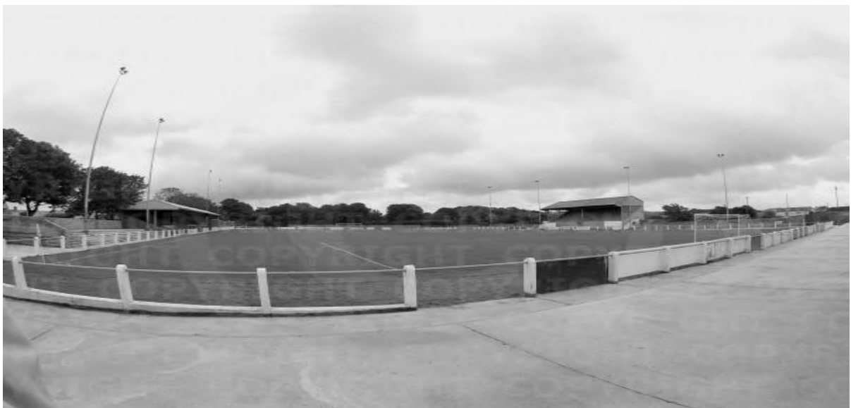
Stair Park old Grandstand Sns
